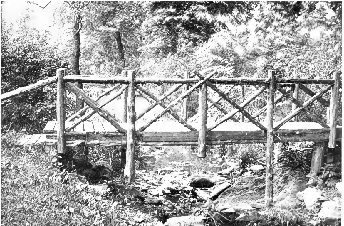
A rustic bridge of extreme simplicity, in keeping with the surroundings, which are as Nature left them.
